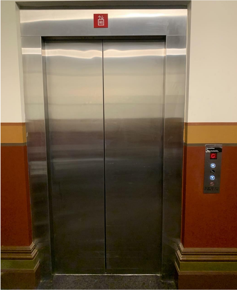
Image description: Doors of the elevator.
